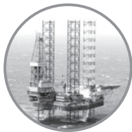
PV DRILLING II
