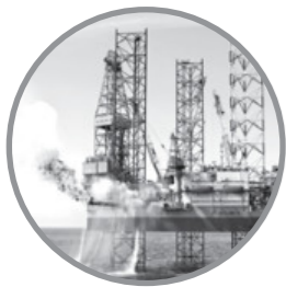
PV DRILLING III
