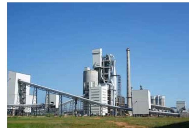
Ha Long cement plant, Quang Ninh
