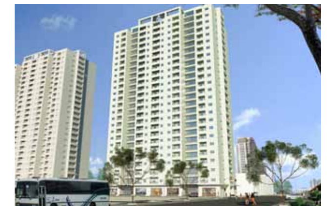
CT2 Building, Van Khe urban, Ha Dong district, Song Da 6, JSC is the investor
